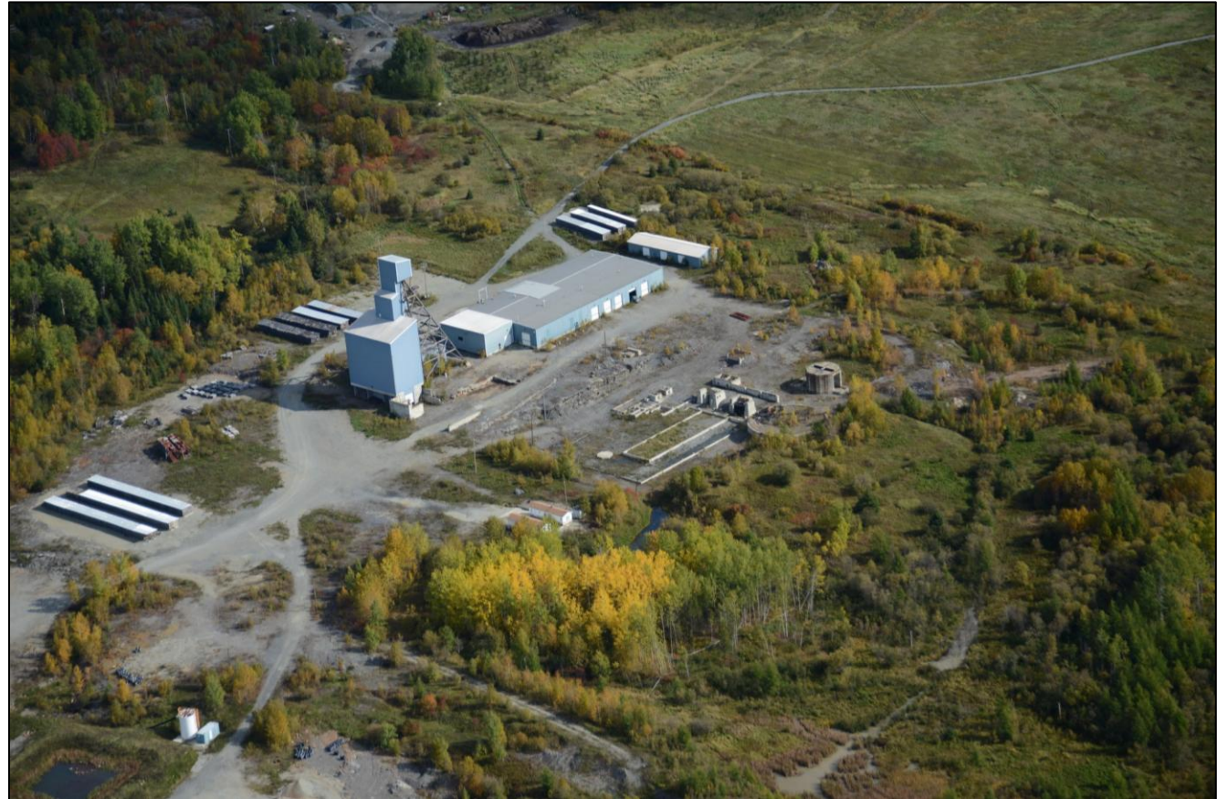
Surface facilities at Rouyn Gold Project, Québec
