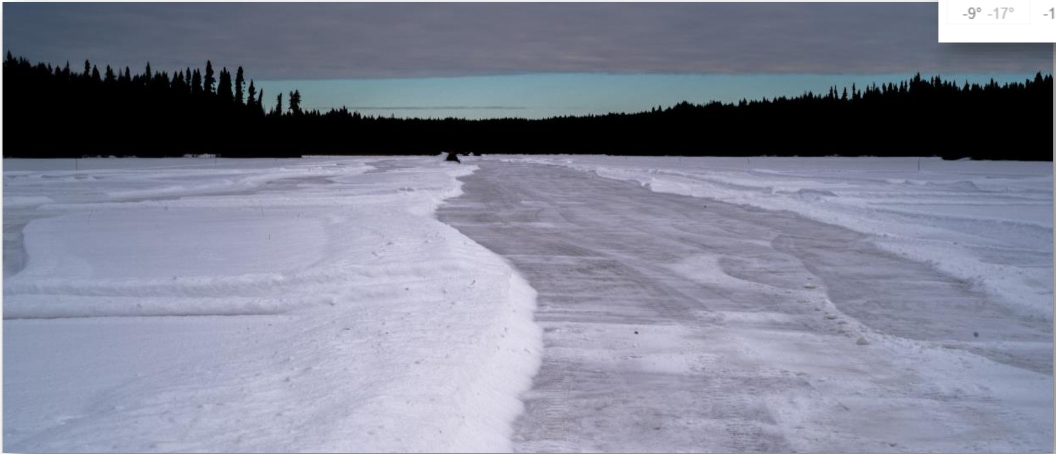
Ice Drill Pad preparation - Kasagiminnis Gold Deposit
