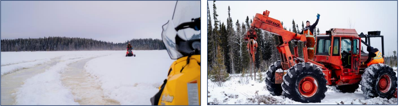
Drill Preparation work currently underway at the Company's Pickle Like Gold Project in northwest Ontario, Canada
