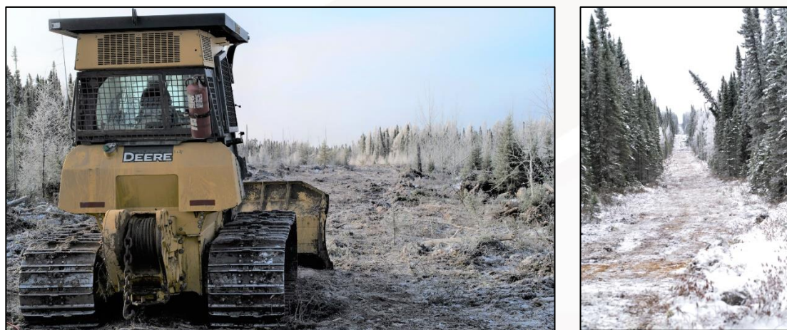
Figure 7 – Construction of Winter Trail to the Kasagiminnis Gold Deposit
