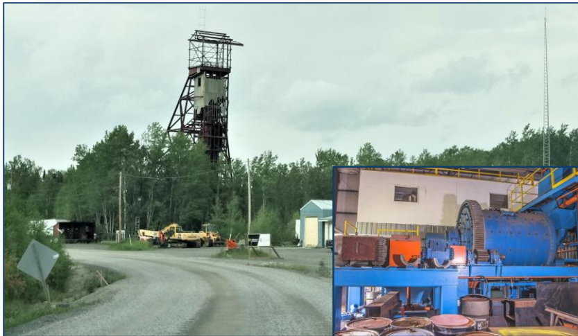
Patricia Headframe and Pickle Crow Mine Plant
