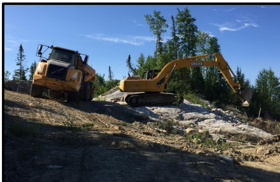
Figure 1. Excavator and truck collecting the bulk sample from North Aubry prospect.
